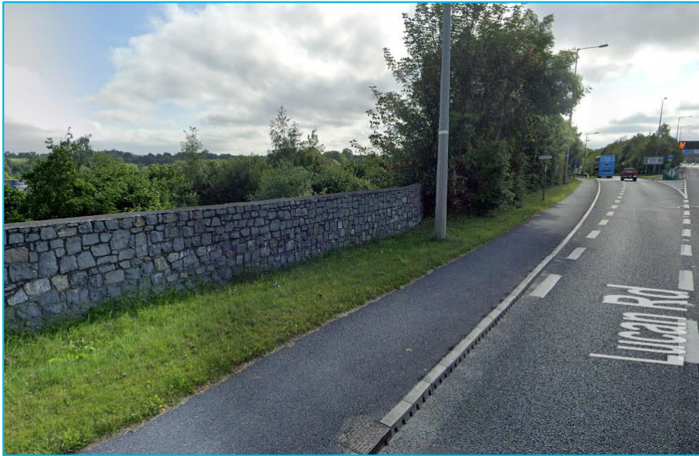
Photo 3 – Proposed retaining wall location looking North East
